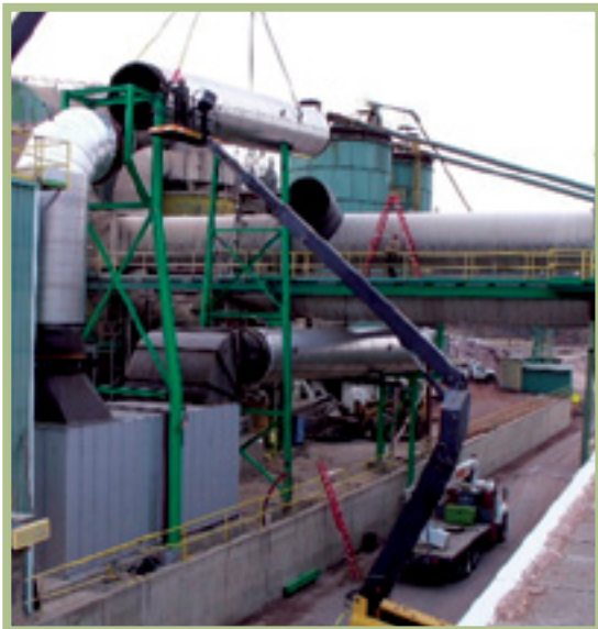
Large Ductwork Design and Installation
